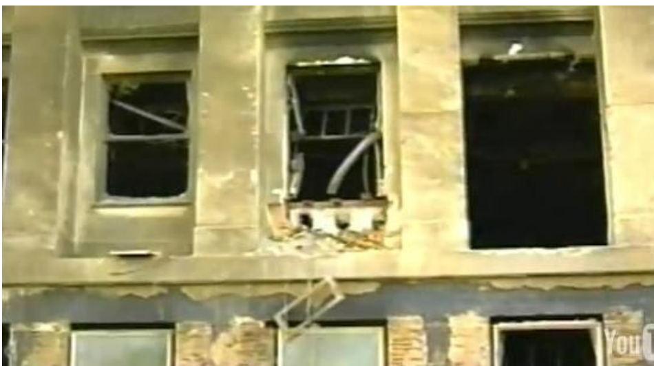
Fig. 5. Left wing impact mark, near horizontal.
